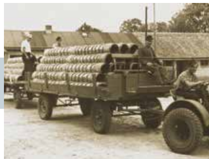
1945 Rebuilding in Knesebeck
