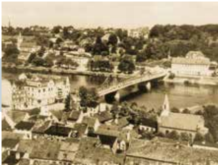
1777 BUTTING foundation in Crossen/ Oder as coppersmith's
